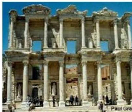
Damage to stonework caused by acid rain at Ephesus, Turkey
