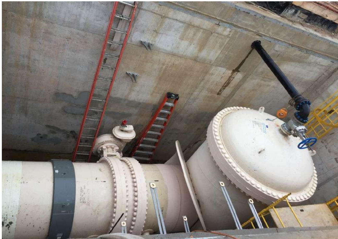
Brooklyn-to-Staten Island Drinking Water Tunnel
