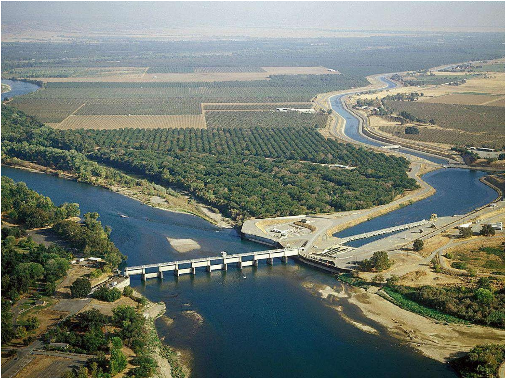
Red Bluff Diversion Dam
