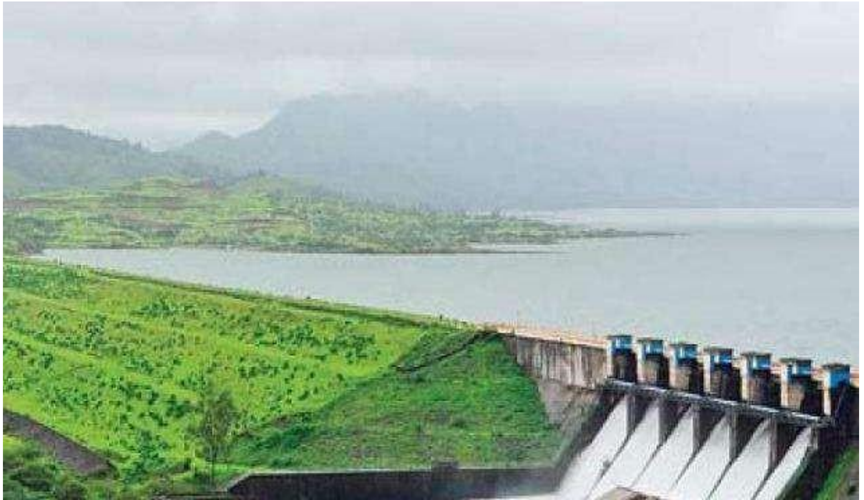
Koyna Dam, Maharashtra
