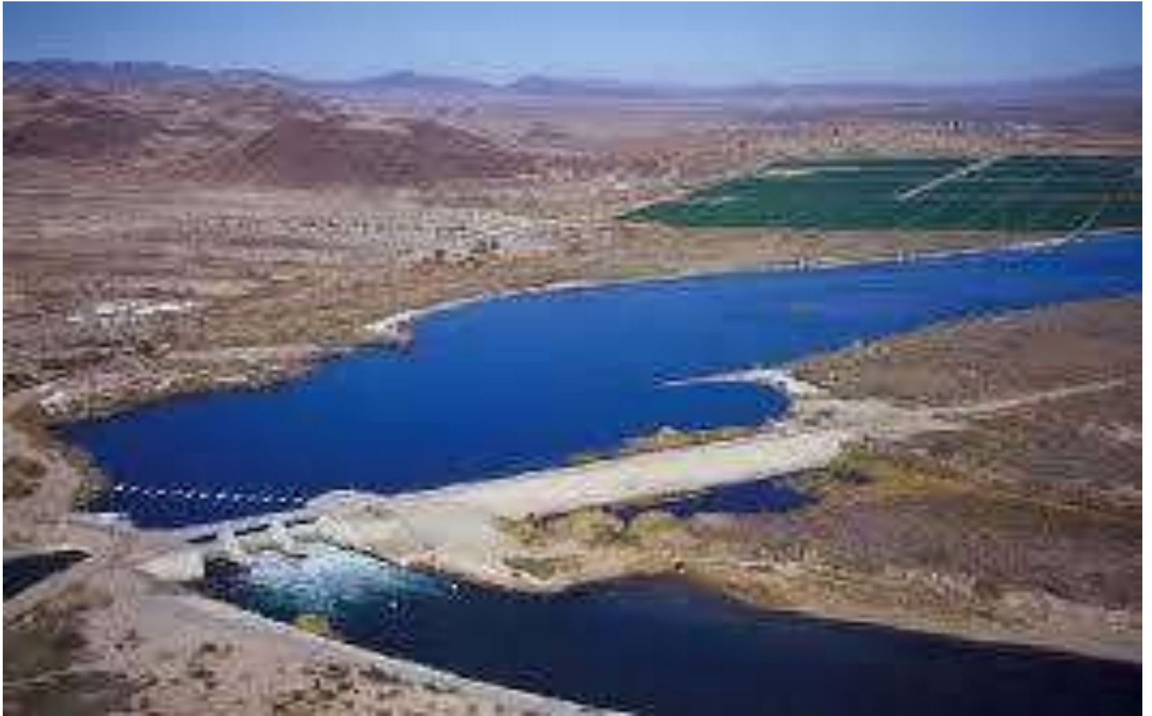
Palo Verde Diversion Dam
