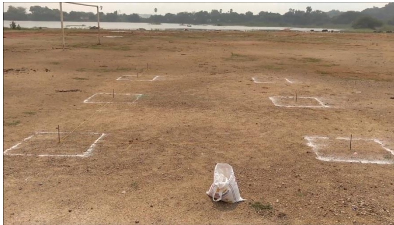
MARKING OF FOUNDATION
